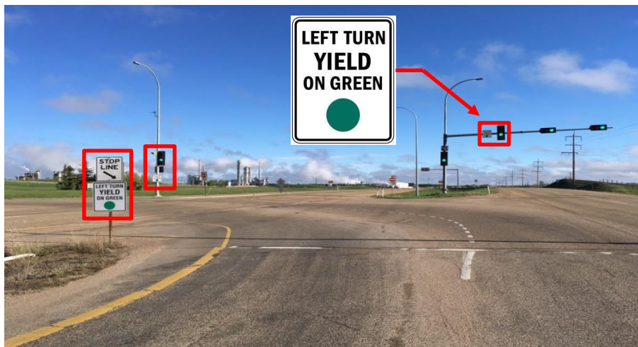
Figure 4 Installation of "Left Turn Yield on Green" signs
