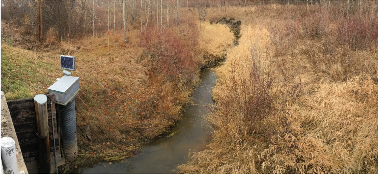
Photo A-21 Pointe-Aux-Pins PAP#6, facing downstream (northwest). Note WSC hydrometric station on bridge, and the bank erosion downstream of bridge (10/30/2017)
