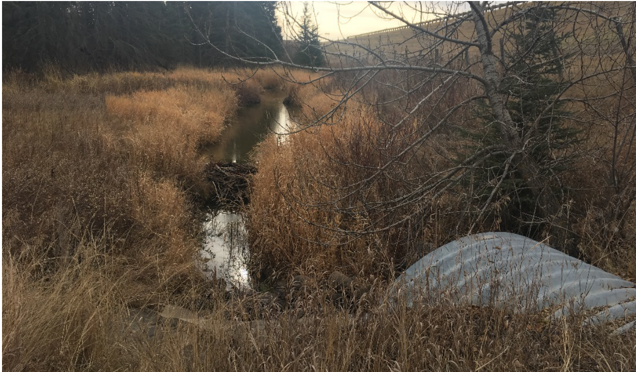
Photo A-13 Pointe-Aux-Pins PAP#2, facing upstream (south). Note beaver dam upstream of culvert (10/30/2017)
