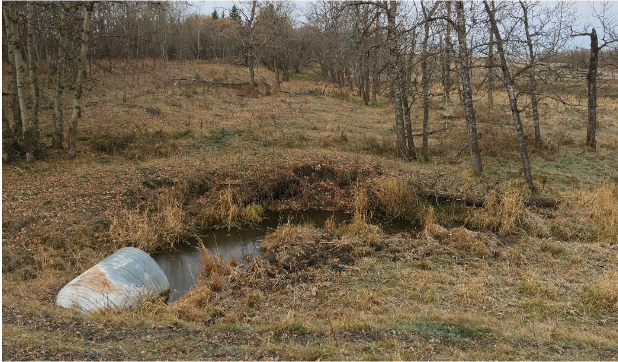
Photo A-5 Old Man Creek OM#3, facing downstream (west). Notice the erosion on the outside bend of creek (10/30/2017)
