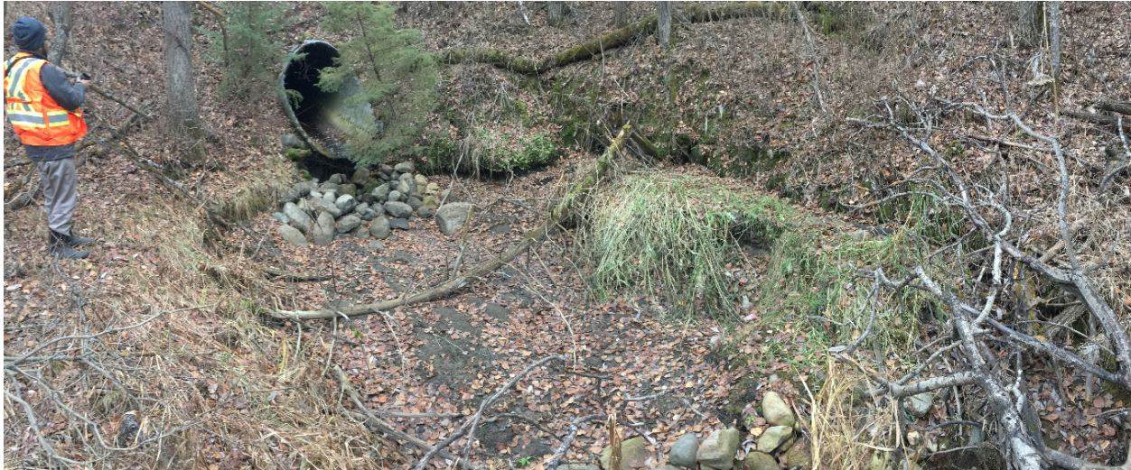
Photo A-23 Pointe-Aux-Pins PAP#7, downstream end of culvert. Large ponded, eroded area caused by constriction in creek on the right of photo (10/30/2017)
