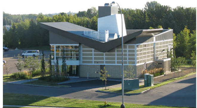
Image 3.2 Strathcona County Community Energy System
