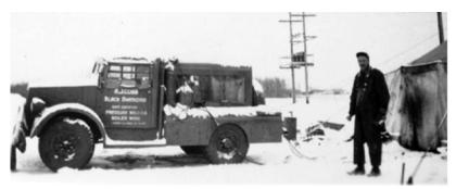
Figure 25. Welding truck constructing two 8-inch lines from Nisku to Devon Field, Leduc, Alberta, circa 1947. Credit: Glenbow Archives / PA-3027-8.
