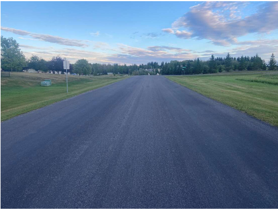
Rural residential subdivision road with hot mix asphalt surface
