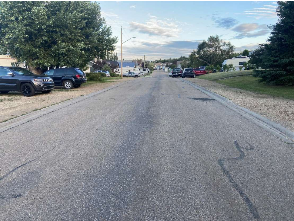
Rural hamlet road with hot mix asphalt surface
