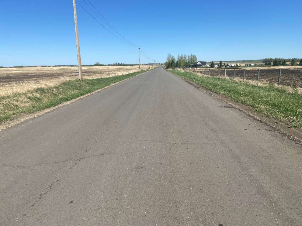
Class III road with new dust abated surface
