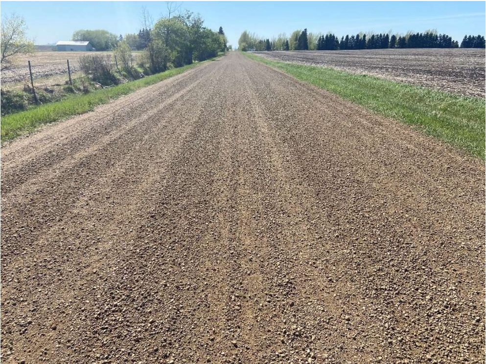
Class IV road with loose gravel surface
